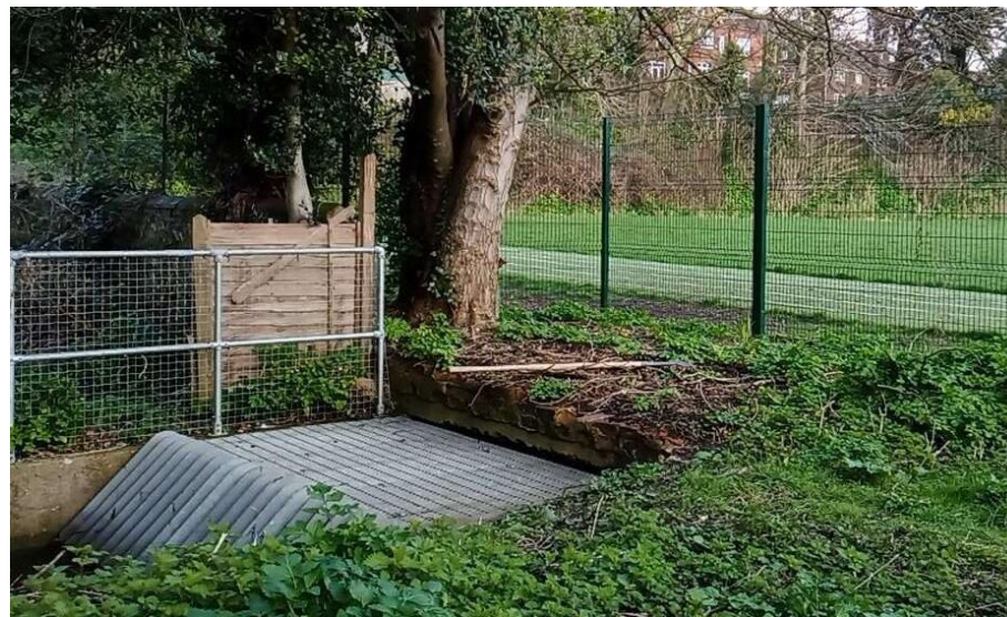
Stream entering Southover School through a trash screen and culvert, potential to daylight this section of the Lewes Winterbourne
