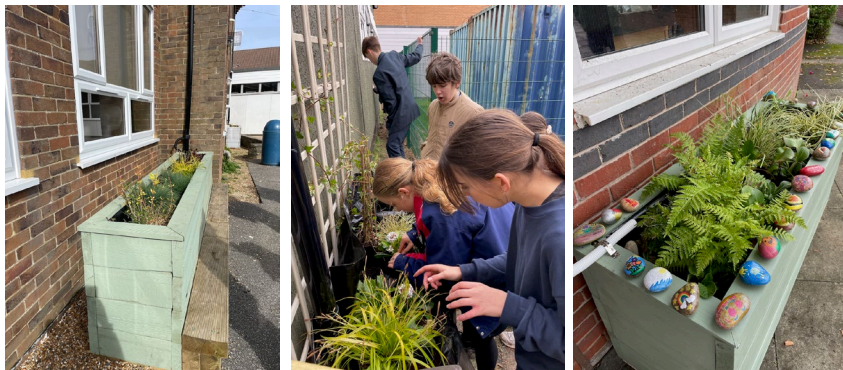
Rainbox planters installed in Ringmer School to slow surface water and engage pupils
