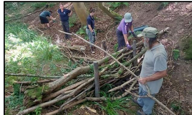
Complimenting the long-term plan, materials have been created (brushwood bundles from waste products of local coppicing) for future use and pilot projects have been delivered to plant trees & cross-slope hedgerows and install leaky dams on pathways which see high levels of surface water during storm events.
