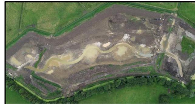
The new channel has been designed to meander through the site and has a shallow profile, enabling both connectivity with the floodplain and resilience against future periods of low flow resulting from climate change impacts. Other works saw a chalk gravel substrate installed at points in the new channel along with the construction of two public footbridges and hydroseeding 4ha of wetland wildflower meadows.
