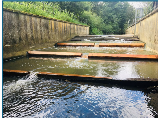
Technical fish pass fitted to Ardingly Gauging Station in 2022 (left) and removal of Buxted Park Weir in 2012 (right)
